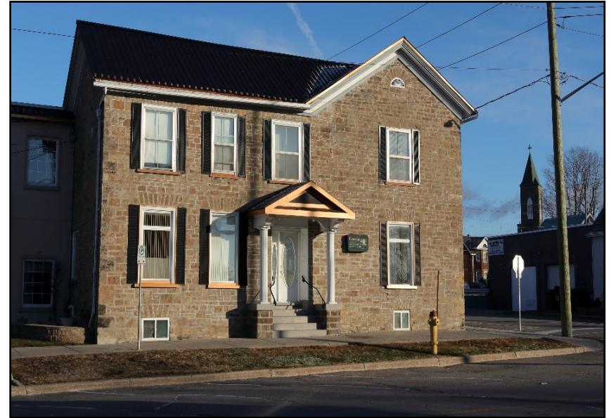
Figure 21: An example of exterior shutters on a 2-storey brick building.
