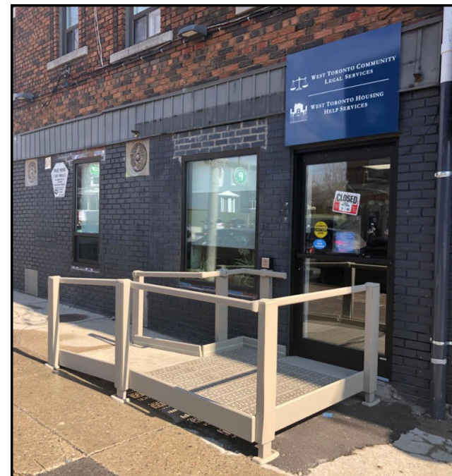
Figure 8: The use of an accessible ramp creates a more inviting environment by providing a barrier-free entrance for all users.
