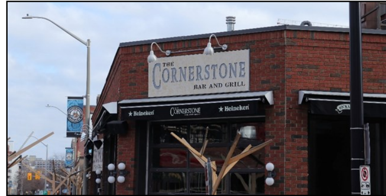
Figure 23: An example of exterior gooseneck lighting on building storefront used to illuminate the façade of the building.
