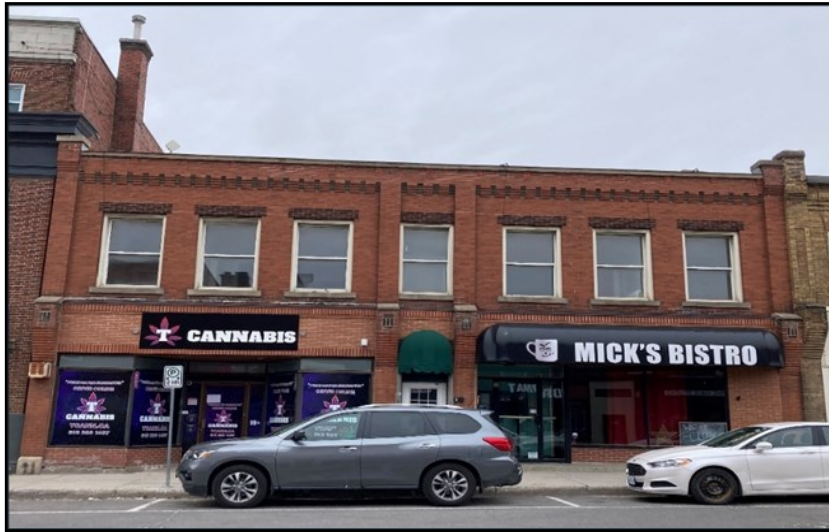
Figure 3: Located at 4 Russell Street East, this building is a great example of Renaissance Revival with its use of corbelling on the second floor.
