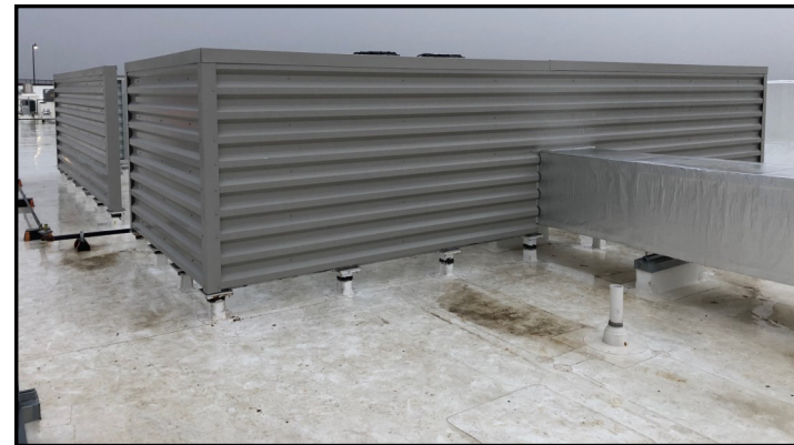
Figure 10: Rooftop screens used to screen rooftop equipment is a great way to incorporate a parapet wall on top of buildings in the Downtown Core as it reduces the visual impact of the rooftop equipment.
