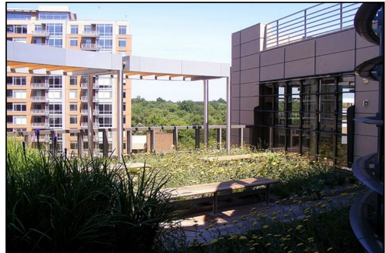
Figure 7: Greenroofs such as the one pictured here is great way to incorporate low-impact development techniques to reduce water runoff, conserve energy and create more urban green spaces.
