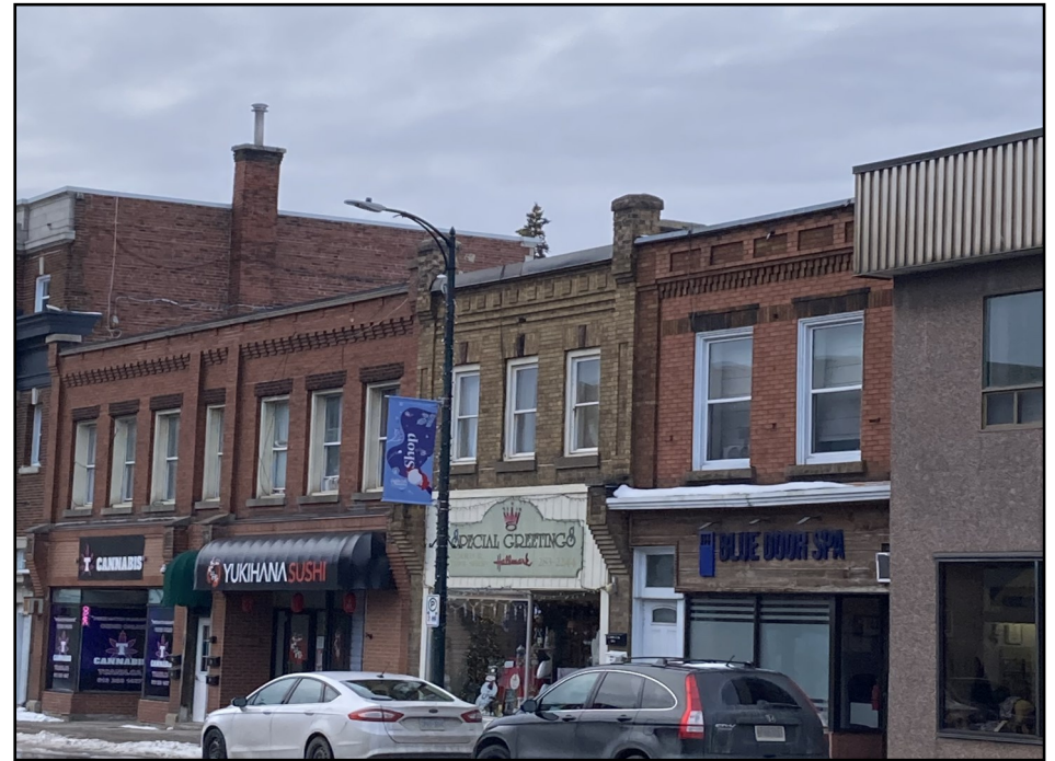
Figure 15: An example of a distinctive roofline created by corbelling along the four buildings. One important aspect to recognize is the consistent height of the buildings which contributes to a sense of compact form, strong street presence and design uniformity.
