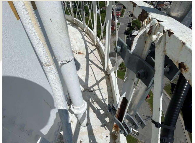
Replace corrodible 'D' rings with stainless steel
